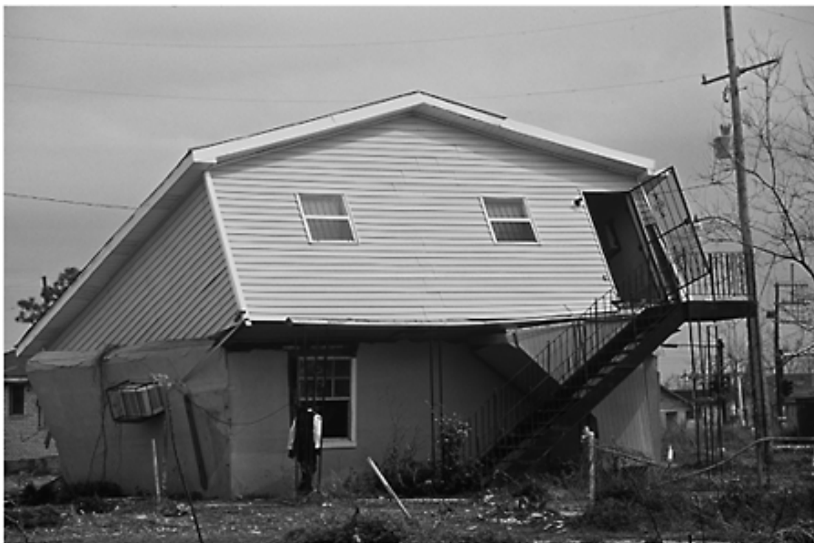
Figure 9.3 New Orleans: One of the houses overturned by a surge of water from the collapsed floodwall of the Industrial Canal during Hurricane Katrina, August 2005.
