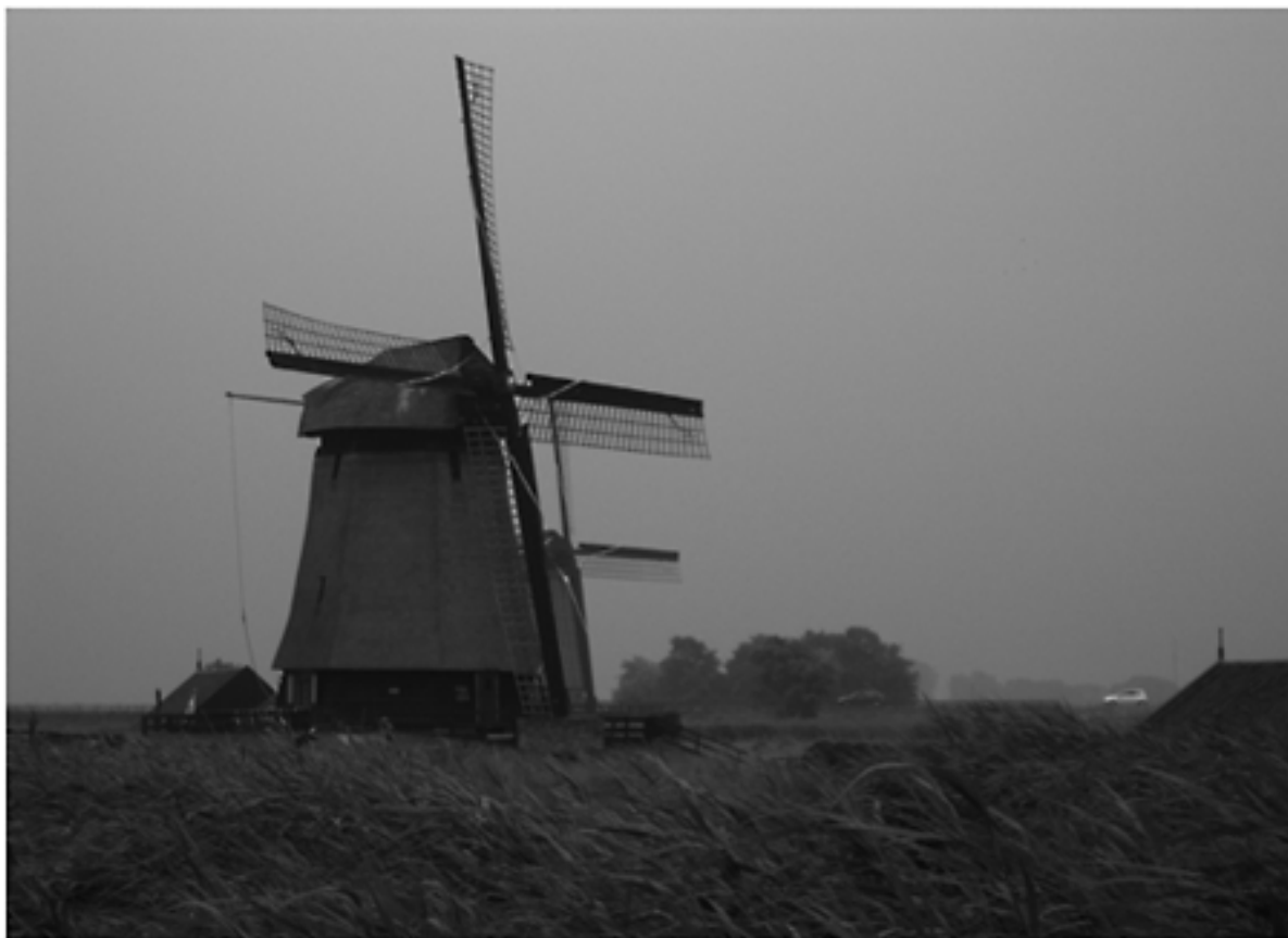
Figure 6.2 Drainage windmills in the Schermermeer polder, Netherlands. These provided energy for machines such as the Archimedes screw pump to raise water into canals and make land available for agriculture. Photograph taken in 2007.
