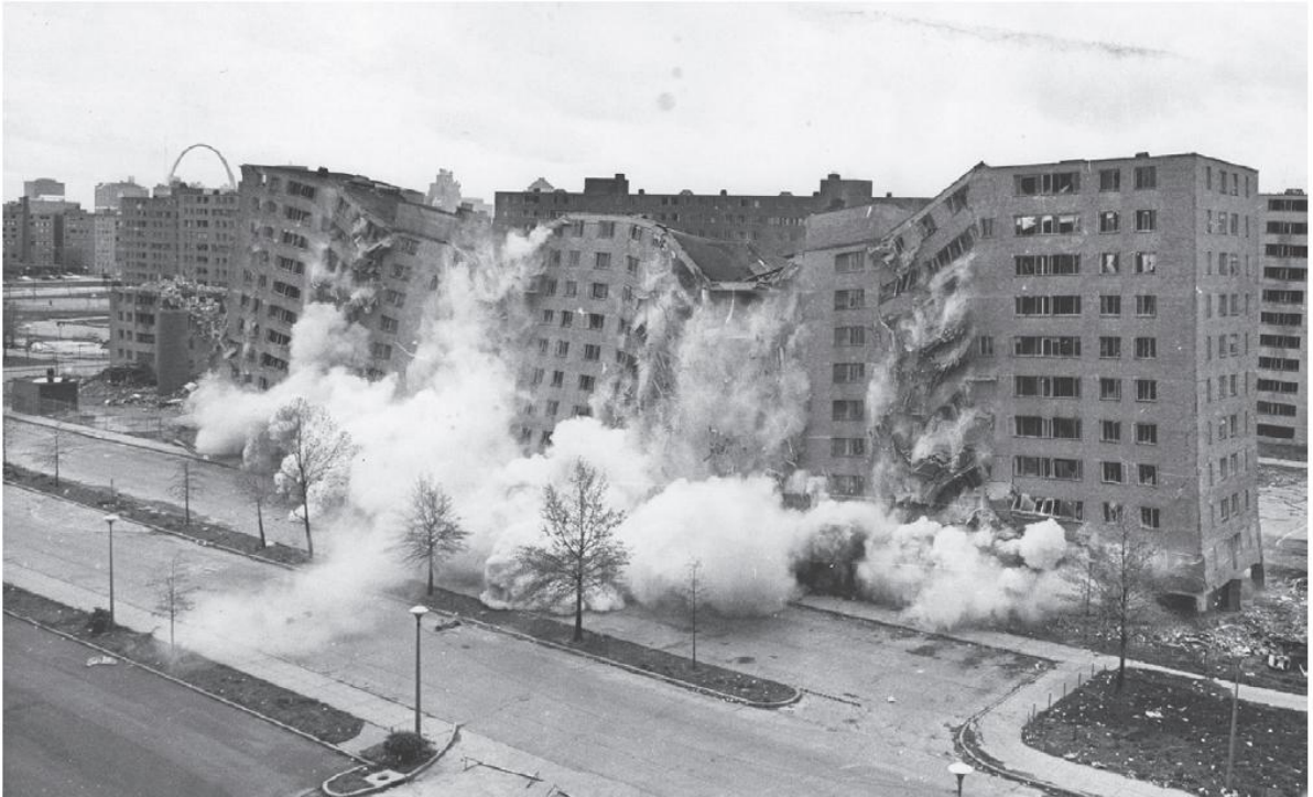
Demolition of Pruitt-Igoe, April 21, 1972, US Department of Housing and Urban Development
