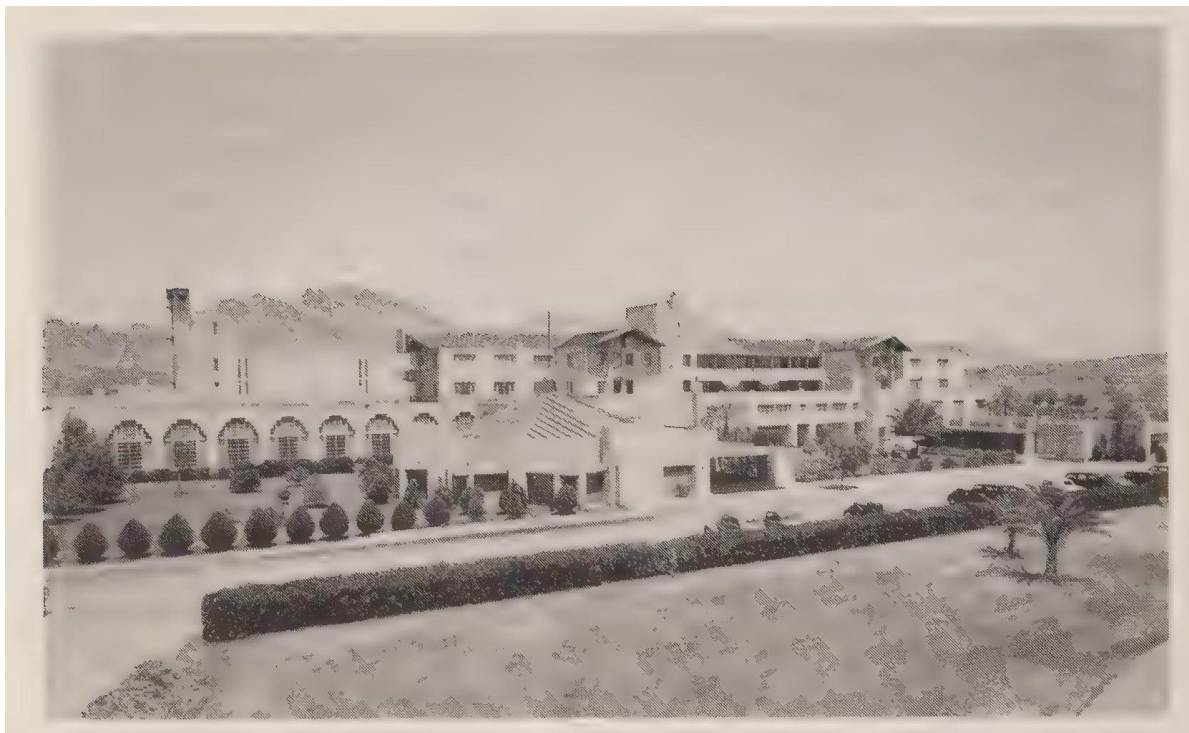
Fig. 5.2. Biltmore Hotel, 1929 (CPSPC108:4 51: courtesy Arizona Biltmore Hotel Photograph Collection, Arizona Collection, Arizona State University Libraries). The Arizona Biltmore offered guests elegant accommodations isolated from both the urban bustle of the city eight miles away and the bristly ruggedness of the desert setting nearby. At the resort guests could experience the desert in recreational venues such as horseback riding. Within the hotel grounds, however, the desert would be banished. The manicured lawn, hedge row, palm trees, and shrubs at the entrance to the resort appeared as a bulwark against the looming desert mountains in the background.
