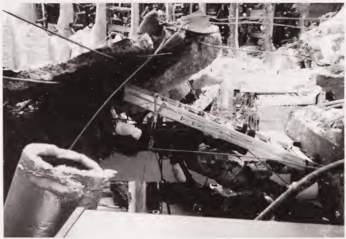
The ruins of the Murrah Federal Building in Oklahoma City.
