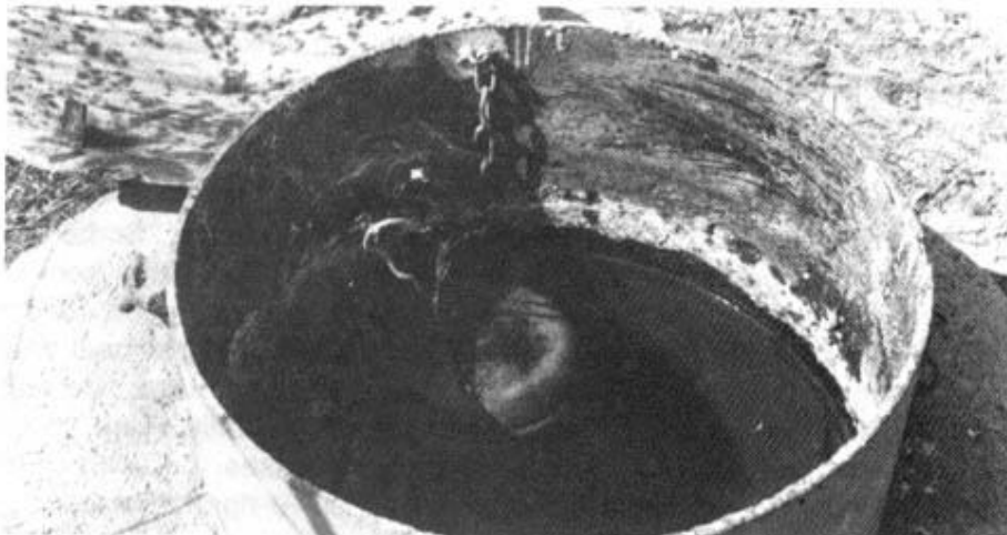
Float-valve regulates water level in stock tank.
