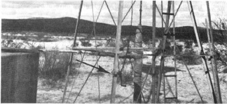
Windmill. Note windlass (arrow).
