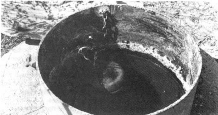
Float-valve regulates water level in stock tank.
